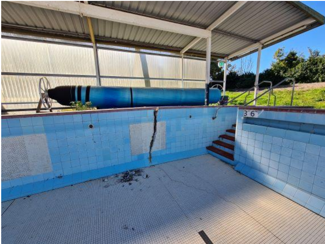
Photo 1: Looking north showing a large crack in the pool wall
